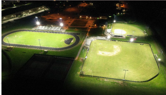
Marshall HS – Field Lighting
